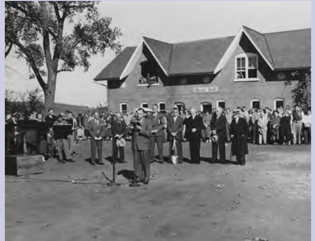
President J.W. Ylvisaker giving a speech at the groundbreaking of Main III, standing outside the Chicken Coop, 1950.
